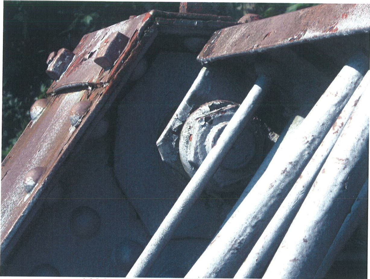
LOG C21-1.00 – U9 TOP PORTAL BRACE CONNECTION
