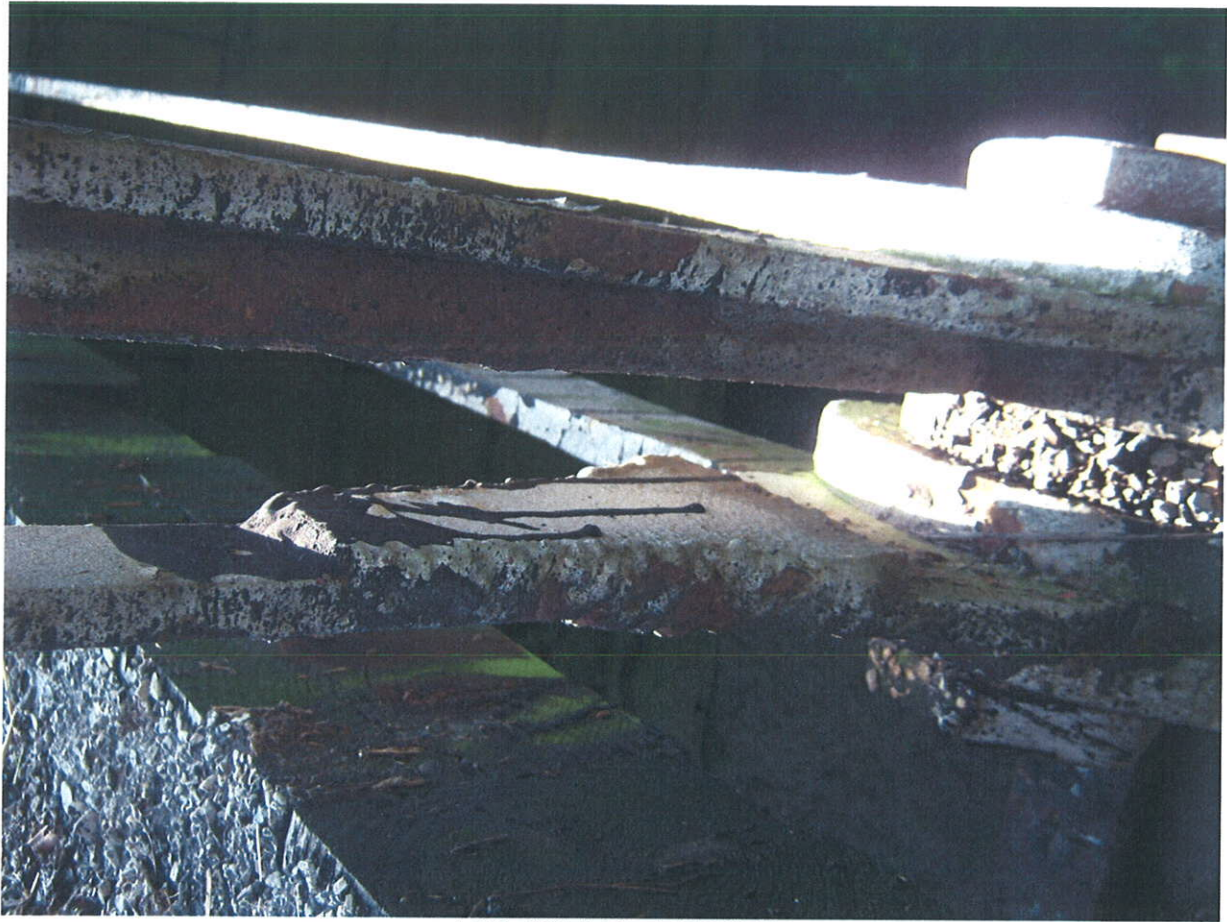
LOG C21-1.00 – L9 REPAIR
