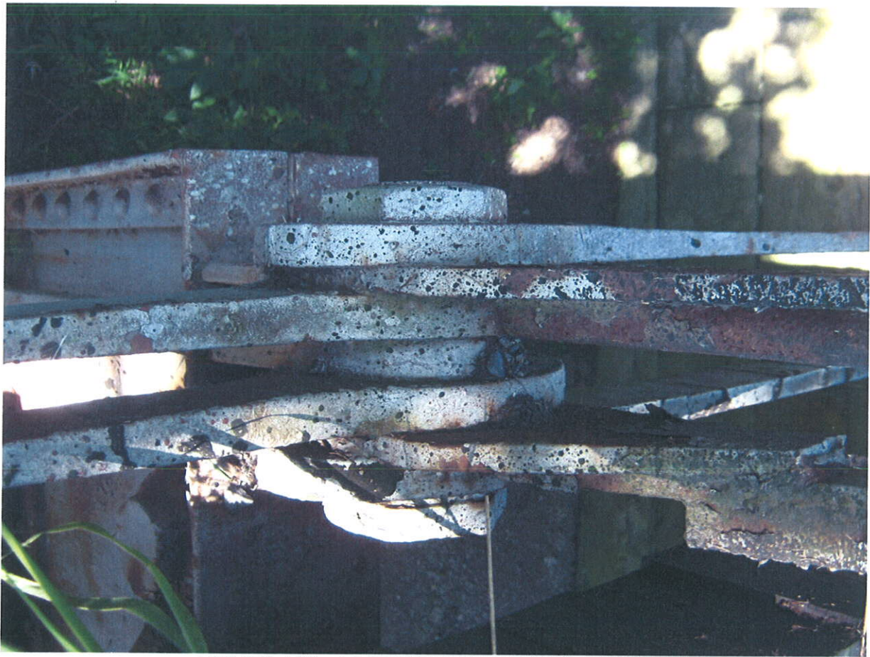
LOG C21-1.00 – L1 REPAIR SOUTH TRUSS (WEST END)
