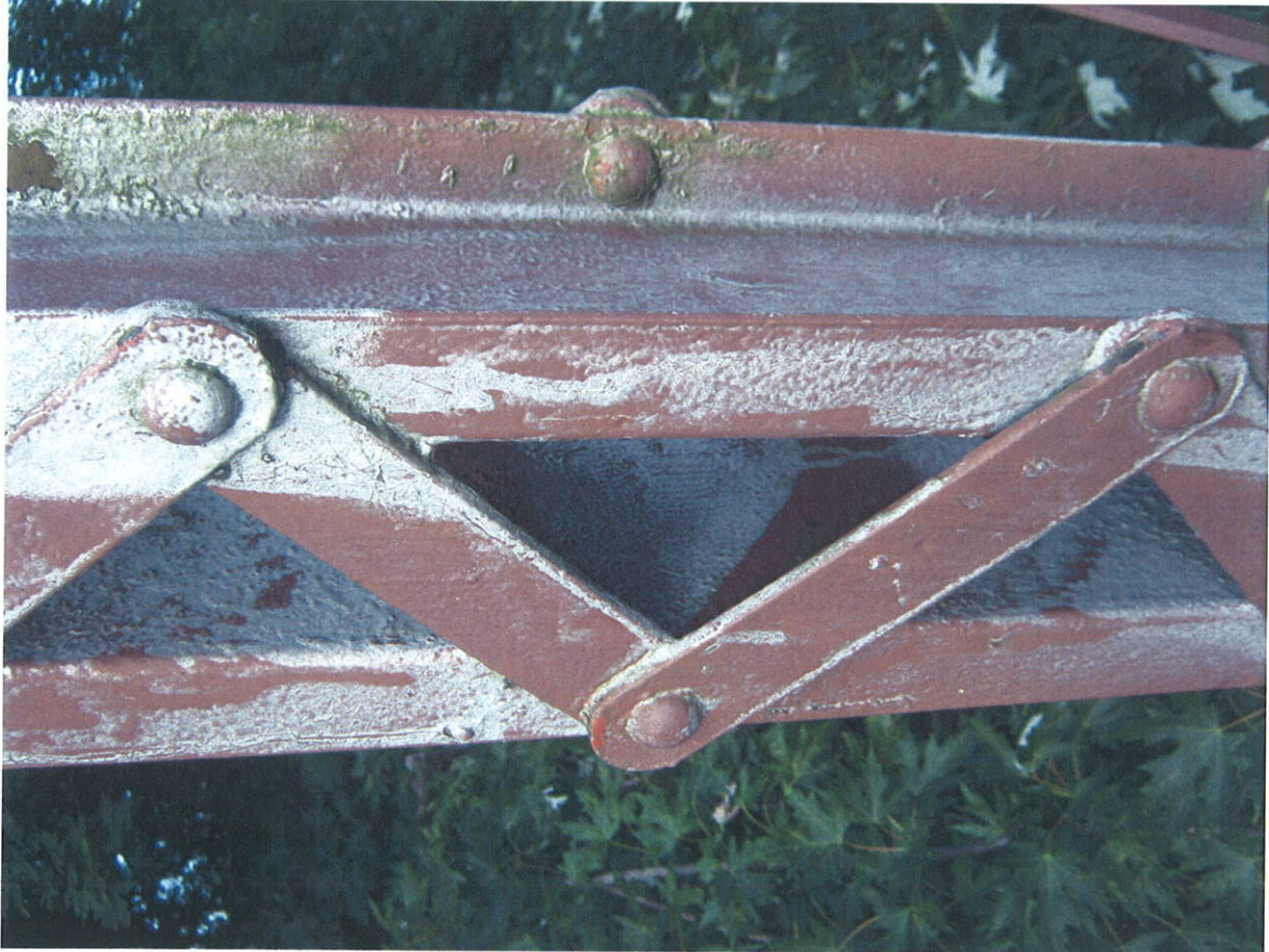
LOG C21-1.00 – TYPICAL VERTICAL LATTICE
