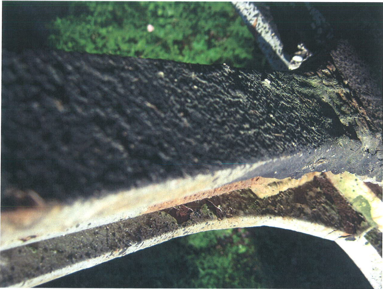
LOG C21-1.00 - L9 REPAIR
